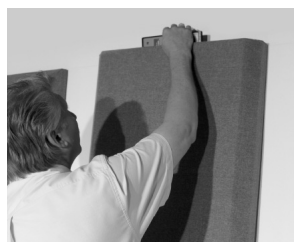
Step 4: Level panel on Set line
