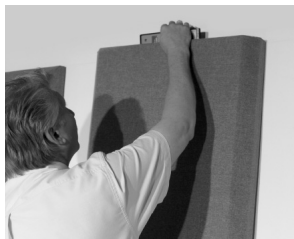
Step 4: Level panel on Set line
