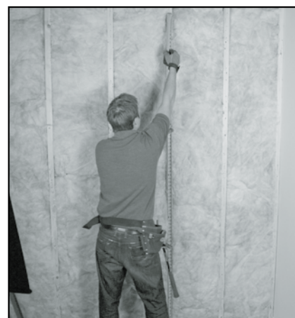
Measure the height of the wall
