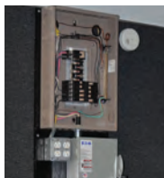
Heavy Duty AC Wiring
