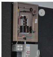
Heavy Duty AC Wiring
