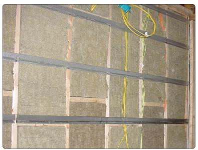
**RC-8's** are specially shaped metal to which gypsum board or other building materials can be mounted to isolate them from the framing members (studs) of a wall or ceiling. **RC-8 Resilient Channel** can add as much as 10 dB of isolation if used properly.
