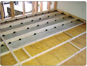
Any size flooring joists (must be 2" nominal – i.e. 1½" wide to fit **U-Boats™**) will work for walls or floors, but again, the larger the air cavity created by the joist, the better the potential decoupling effect.
