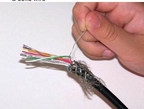
1.8 Fan the wires out into two group base on color coding on page 1
