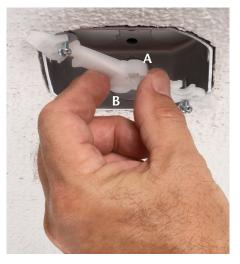
2 Use the bracket opening that works with the ceiling condition: 'A' for flat ceilings, 'B' for uneven or textured ceilings
