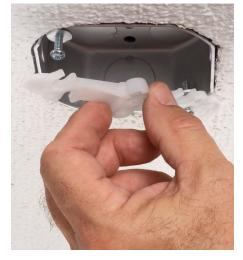
1 Attach the bracket to the box with #8 or #10 screws. Back the screws in the box out just enough to slip the bracket on.
