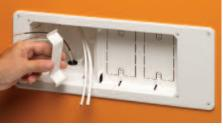
4 Install low voltage separator if using low voltage in double-gang box.
