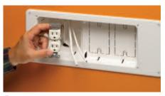
5 Install power and low voltage wiring devices.
