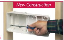
Mount box section to stud through the slotted holes in box. Use minimum of (2)  $\#6 \times 1-5/8$ " wood screws. Positioning tabs place box properly for 1/2 " finish wall thickness.
