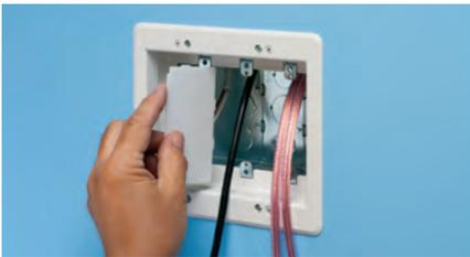
3 Install voltage separator for power and low voltage.
